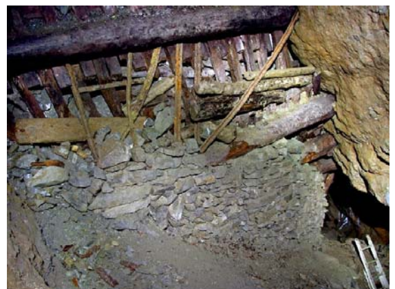
After: Finished repair with pack-wall support
