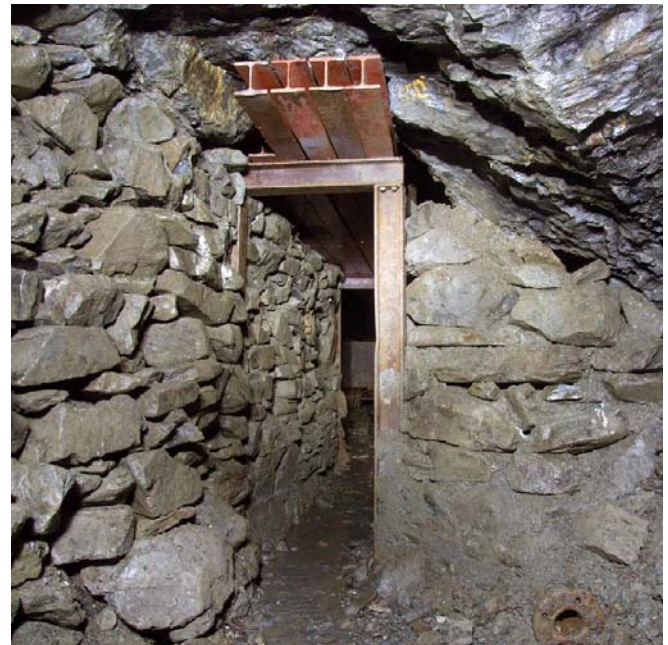
After: Looking inbye to the new steel roadway
