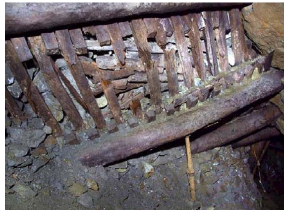
Before: Stull timber with a temporary prop
